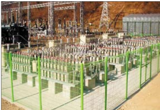
《Harmonic Filter Bank 22.9kV 63Mvar – Doosan Heavy Industrial, Korea》
