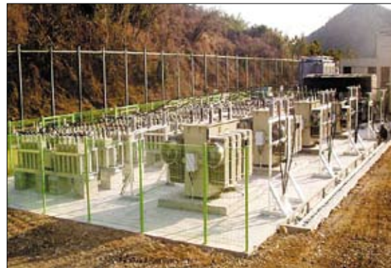
《Harmonic Filter Bank 22.9kV 63Mvar – Doosan Heavy Industrial, Korea》
